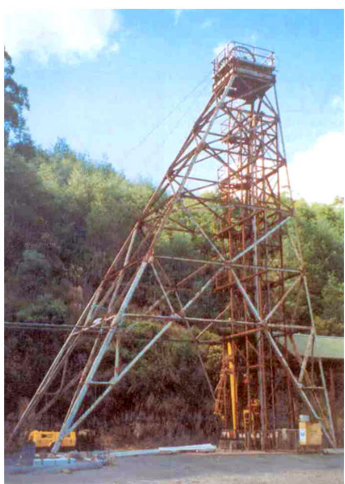
The Morning Star headframe from the Rossarden mine in Tasmania is the focus of a current shaft dewatering and rehabilitation program to gain access down to about 500m.
